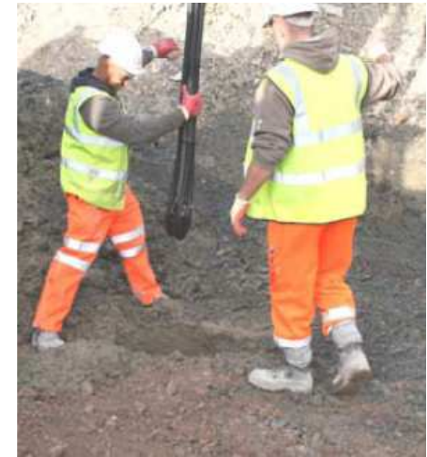
Plunging used T32 bar + 4 pipes (2 loops)
