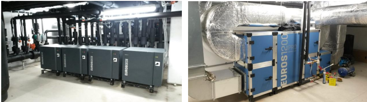
Figure 4 – The heat pumps and the ventilation system located in the basement of the factory.
