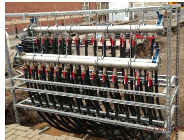
Alternative Wall mounted Sub Manifold
