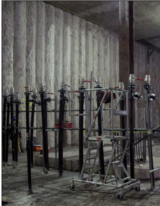
Main flow returns to piles in Plant room
