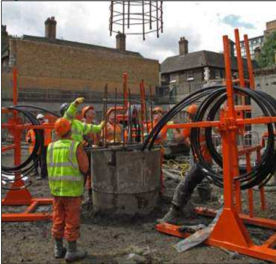
Fixing the loop protection in situ
