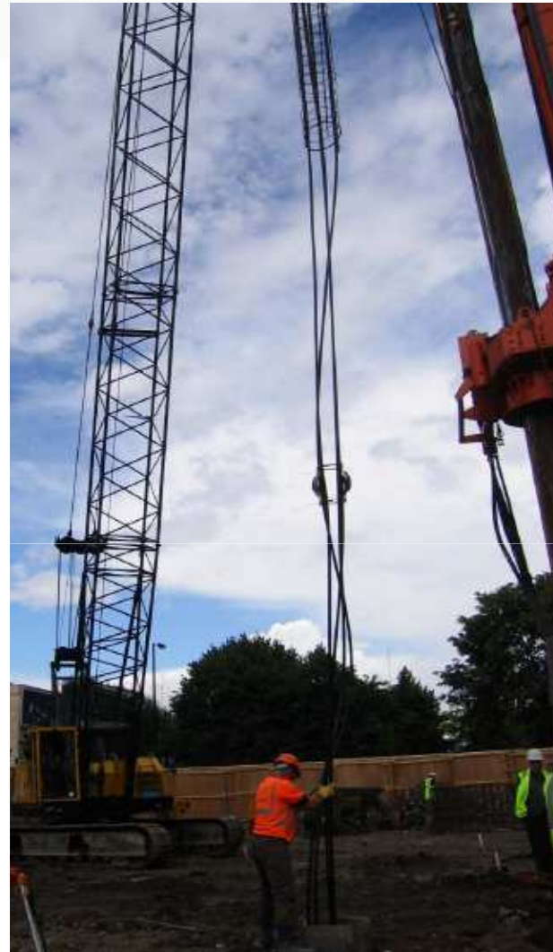
Installation of Geothermal Loops into 25m deep 900mm Rotary Bored Piles at Westminster Academy
