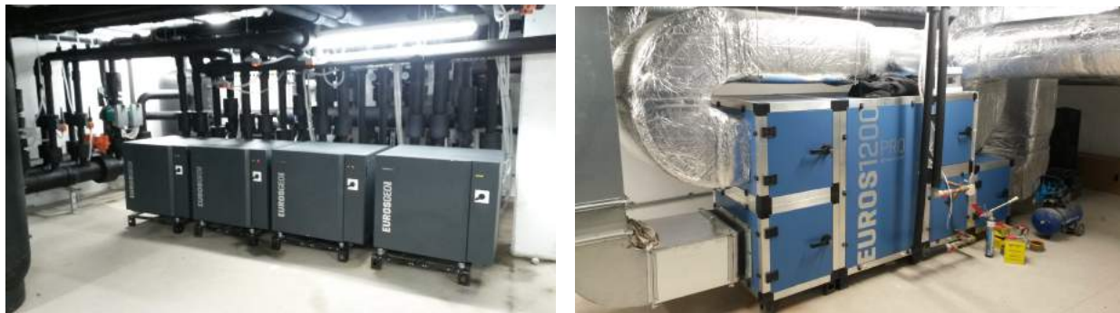
Figure 4 – The heat pumps and the ventilation system located in the basement of the factory.
